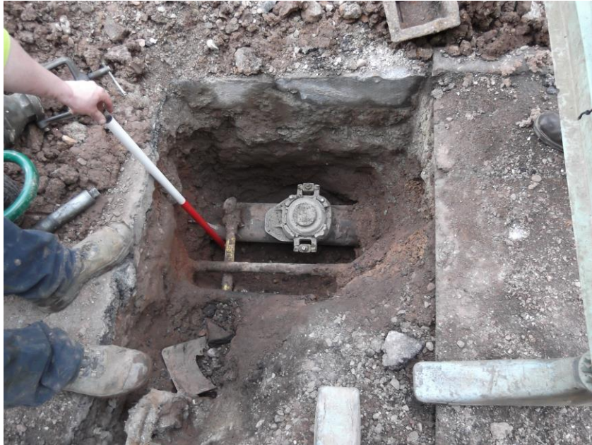
Stonework in the road outside No. 16 Monk Street
