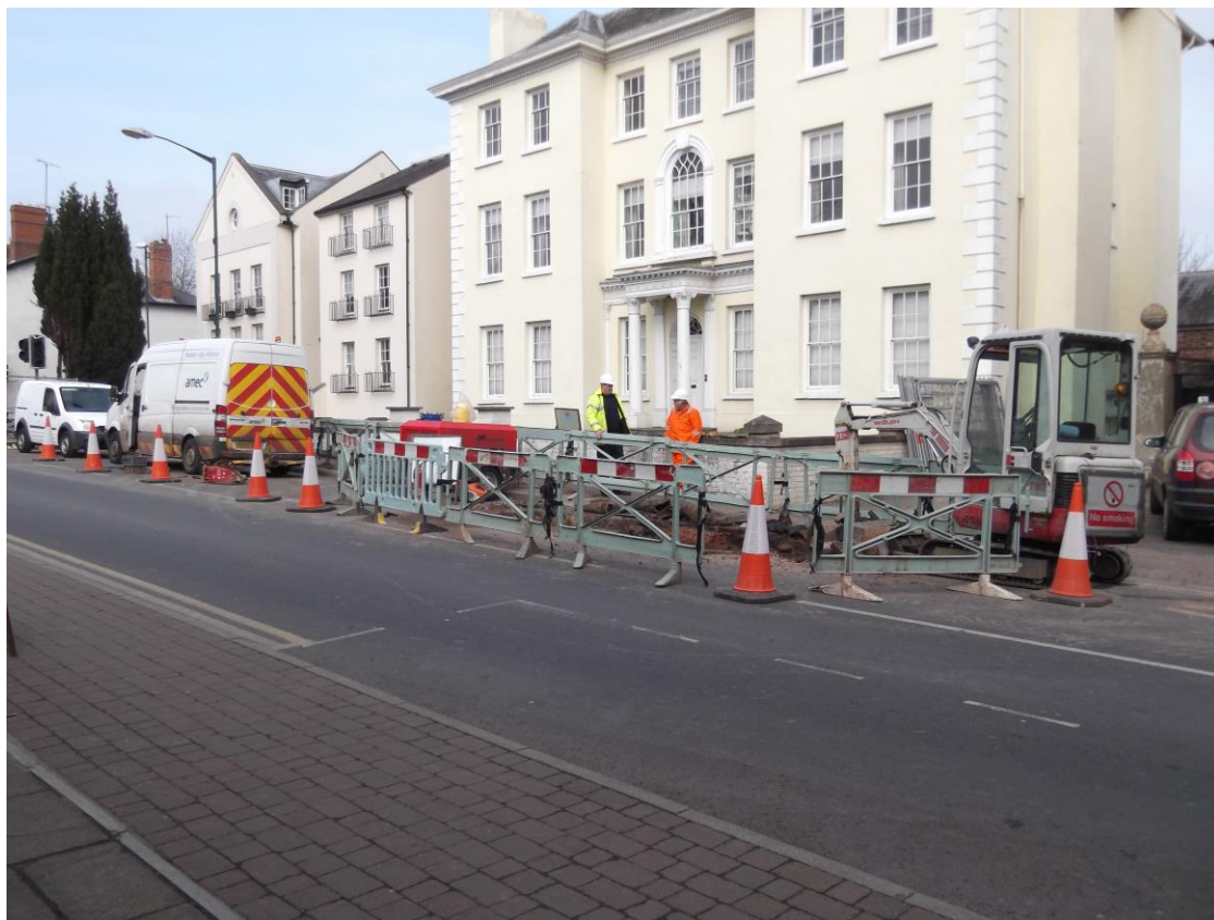
Excavations outside Royal George (1-6 Monk Street)
