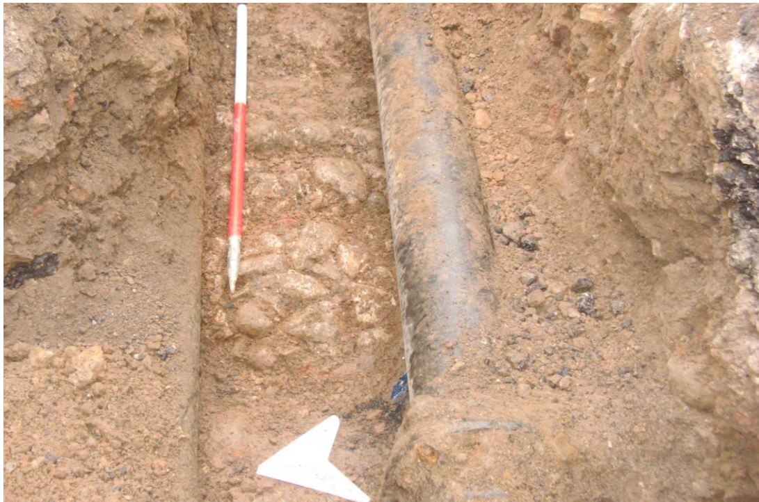
Excavation on north-western corner of traffic lights (SO 50943 13083)
