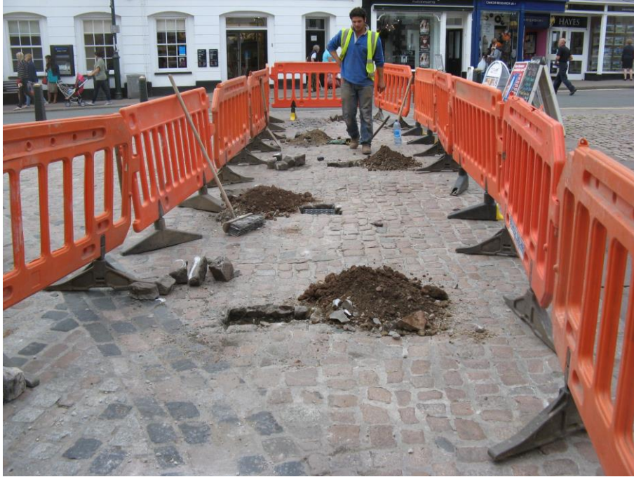
Excavations on the east
